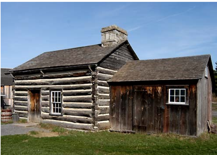
Photo taken by Shannon Kyles of Log Cabin in Upper Canada Village
